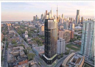
At Wellesley and Sherbourne, 159 SW will include lockers and a repair depot for bicycles, all geared to attracting residents who commute by bike.
