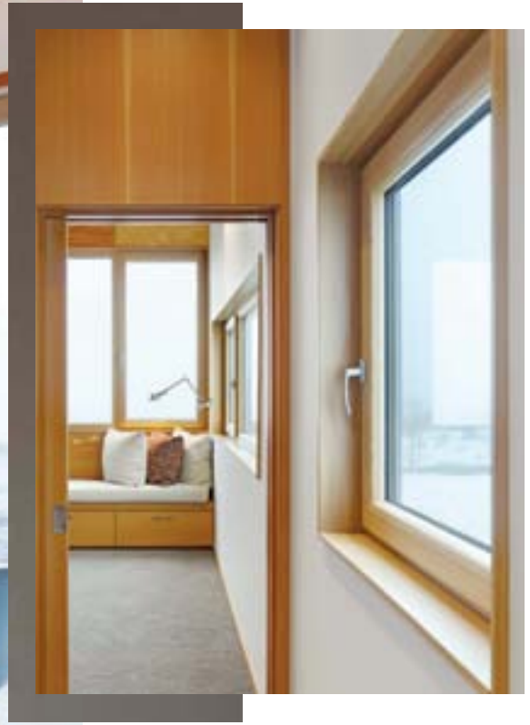
above Douglas fir rift-cut veneers feature on doors and inlaid panels above; the material is also used for interior window frames
